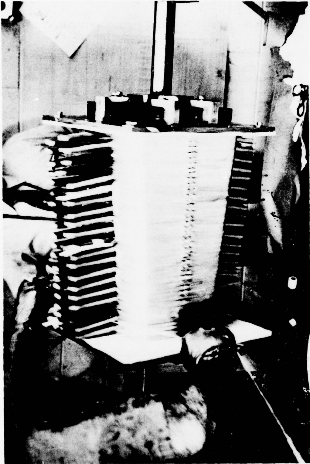
Figure 169. Filament Winding Operation.
