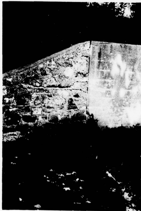
SPILLWAY AND APRON (Looking West)
