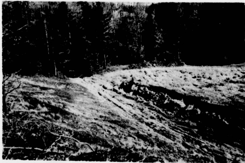
VIEW OF DOWNSTREAM END OF SPILLWAY LOOKING EAST
