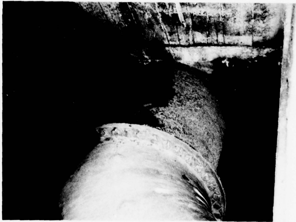
PENSTOCK SECTION THROUGH DOWNSTREAM FACE OF DAM. ROUGH EDGE ALONG RIGHT SIDE OF PENSTOCK INDICATES EXTENT OF CORROSION.
