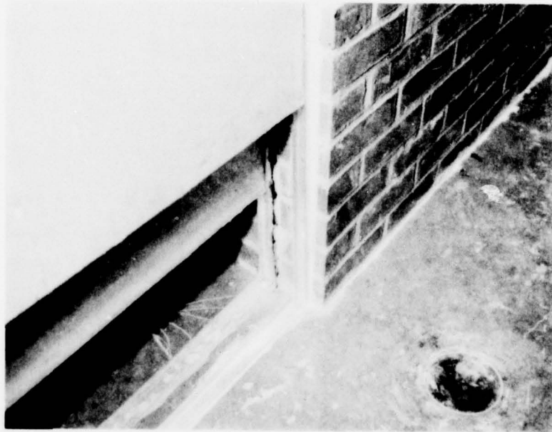
Figure 15. Two sheets of plywood used to form a closure
