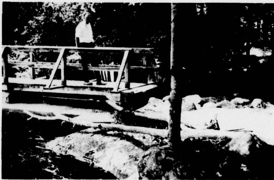
FIGURE 5 RIGHT ABUTMENT (UPSTREAM)
