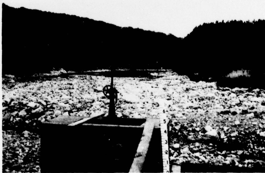
FIGURE 12 DETENTION BASIN AND CONTROLS DOWNSTREAM FROM LAKE KANAWAUKE DAM
