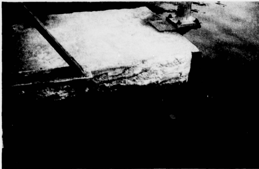
FIGURE 4 SCALING OF CONTROL GATE PLATFORM
