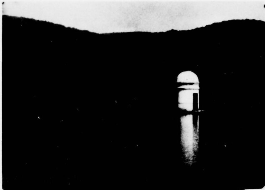
RESERVOIR AND CONTROL TOWER
