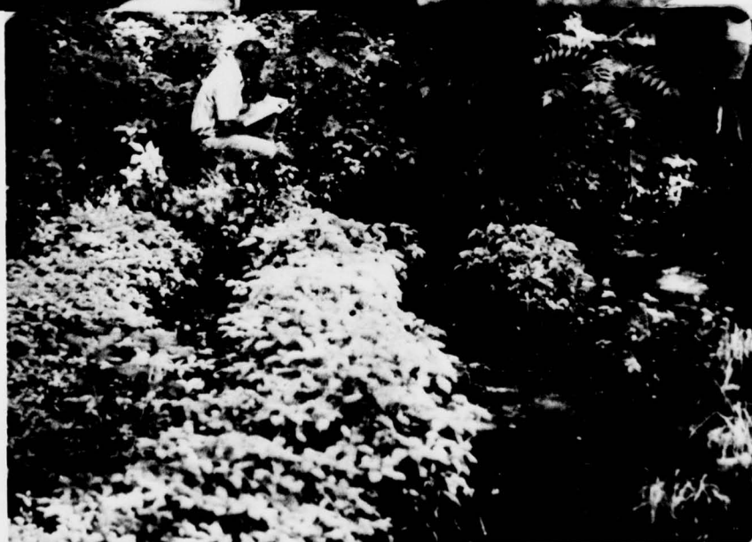
'LEAKAGE' AT TOE OF DAM
