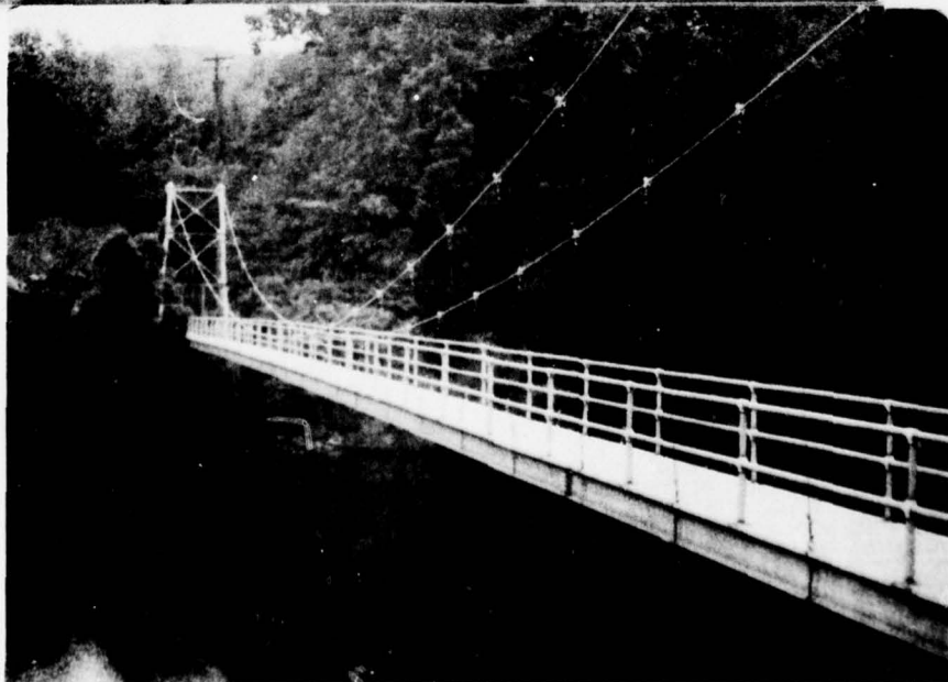
Bridge To Intake Tower
