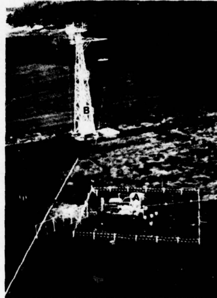
Fig. 1 - Station for triggering lightning (photo EDF).
