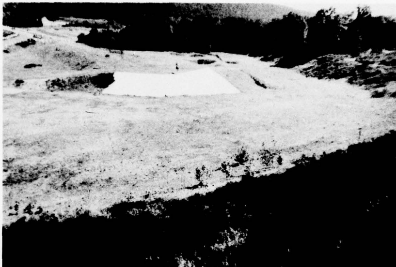
I. Spillway Channel. View from the Right Hillside.
