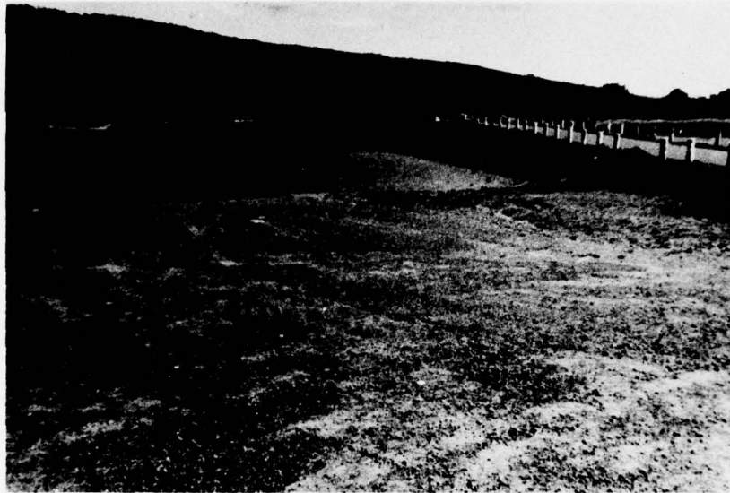
A. Upstream Slope of Embankment. View from Spillway Approach Channel.
