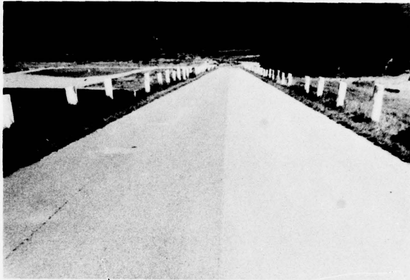
C. Embankment Crest. View from Center of Dam.
