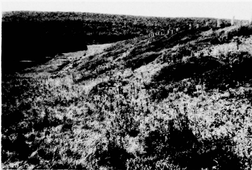
E. Downstream Slope of Embankment. View from the Left Abutment.
