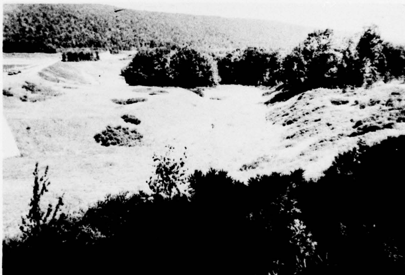
J. Spillway Outlet Channel. View from the Right Hillside.
