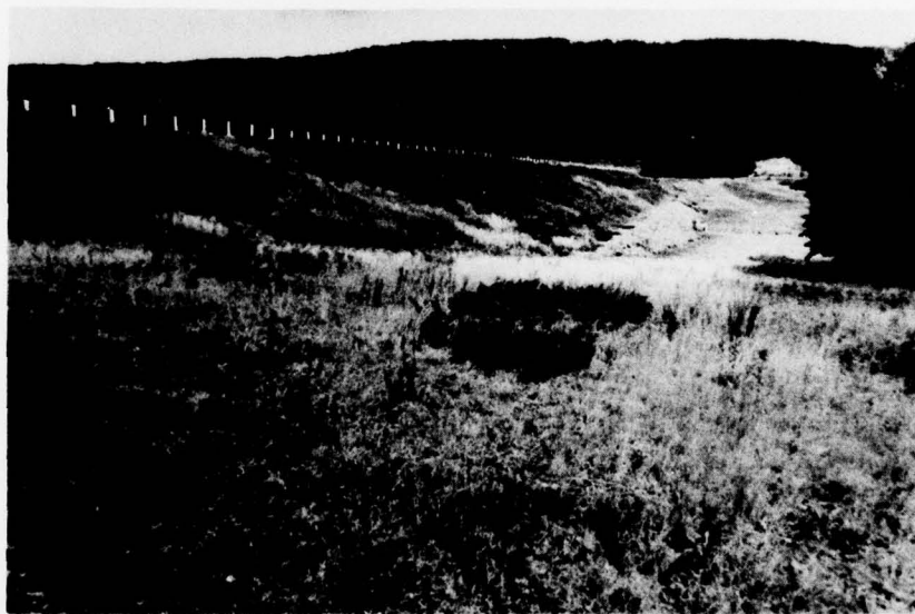
D. Downstream Slope of Embankment. View from the Spillway Outlet Channel.
