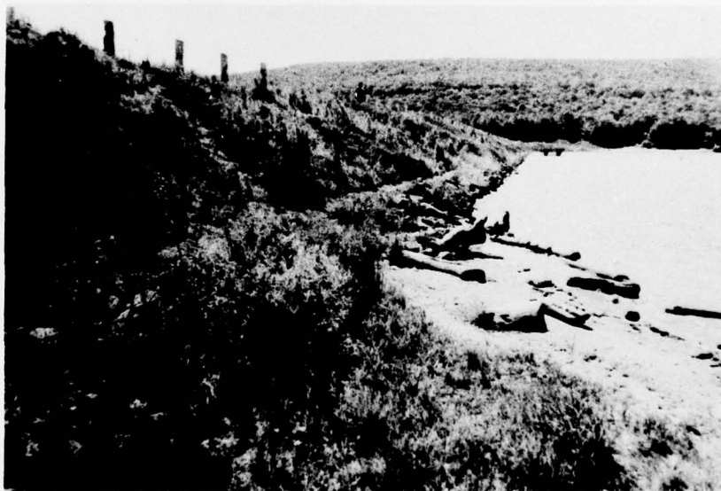
B. Upstream Slope of Embankment View from Left Abutment.
