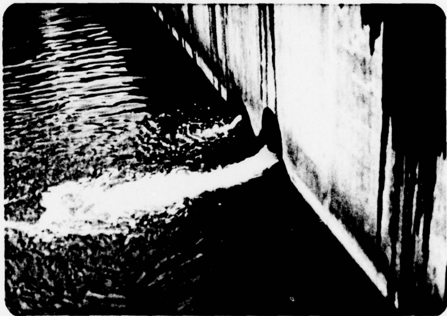
Photograph No. 8 Blow-off pipe discharging.
