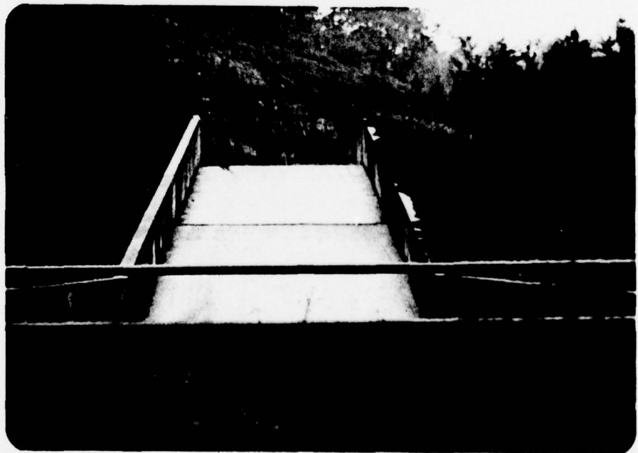
Photograph No. 4 Spillway chute.
