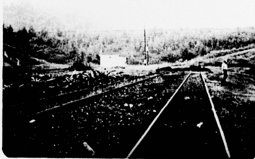
Photograph No. 6 Valve and pump house at the toe of the dam.
