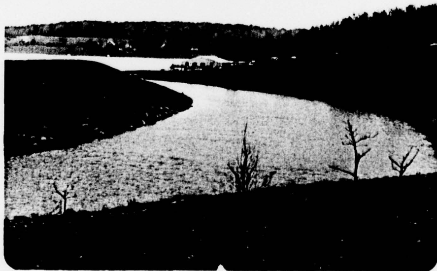
Photograph No. 5 Spillway approach channel.
