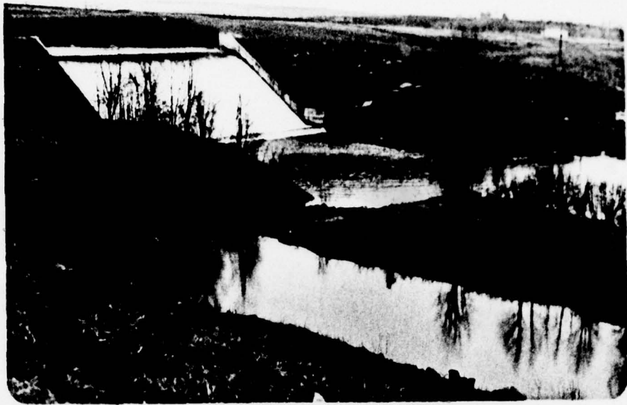
Photograph No. 5 Spillway and plunge pool.
