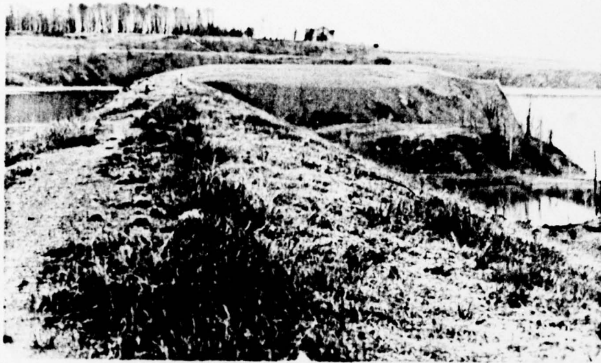
Photograph No. 1 Dam crest.
