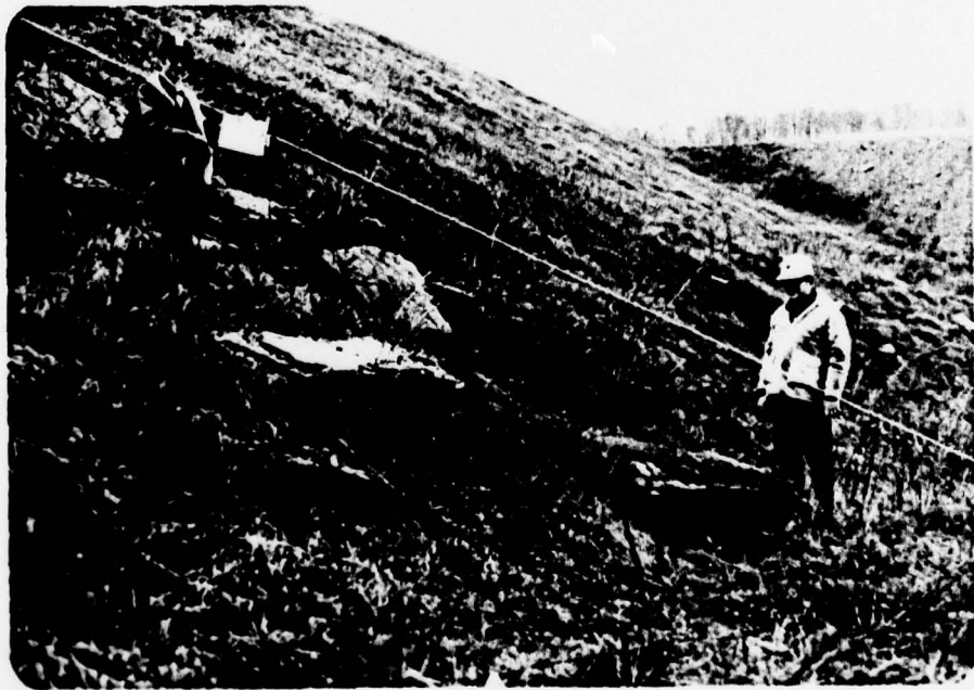
Photograph No. 10 Dam downstream slope irregularity near center.
