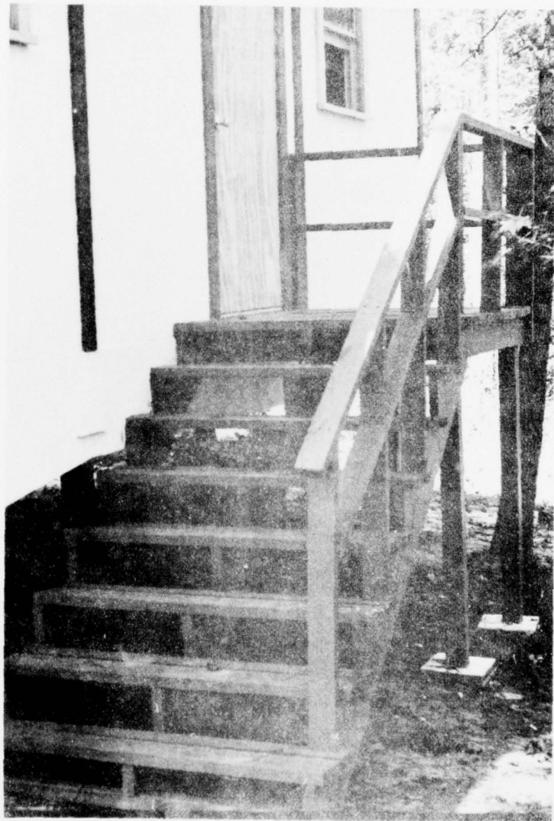
Figure A11. Completed stairway at rear of building.
