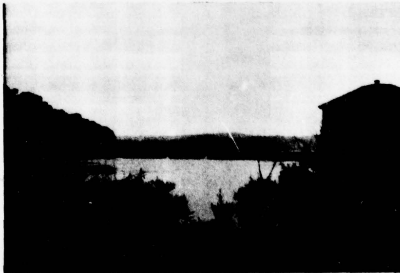
4. View from below dam.
