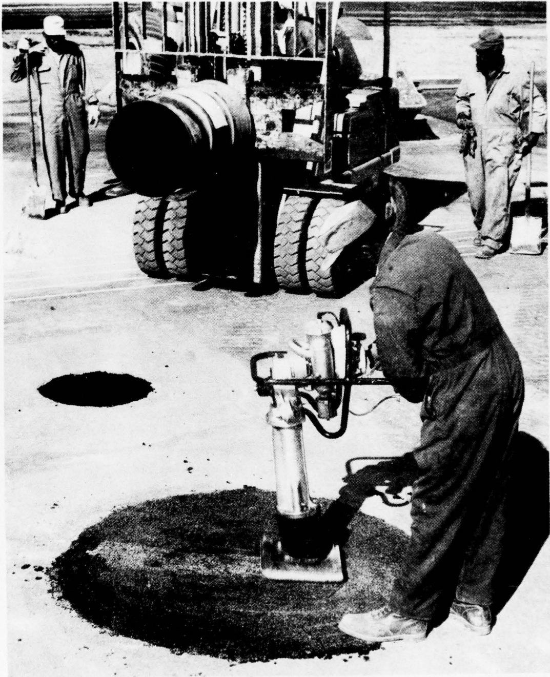
Figure 17. Compacting Zor-X
