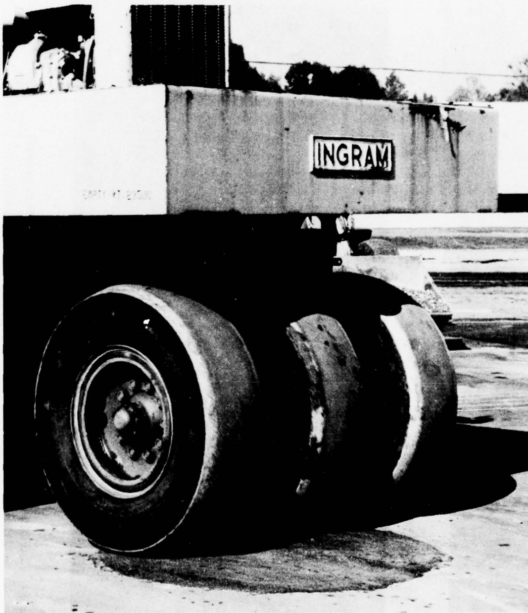
Figure 18. Compacting Zor-X with Pneumatic-Tired Roller
