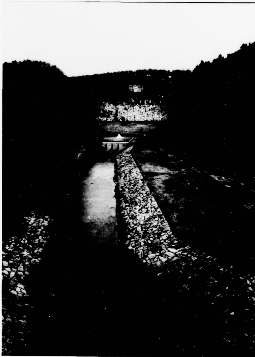
OVERVIEW OF MASONRY DAM
