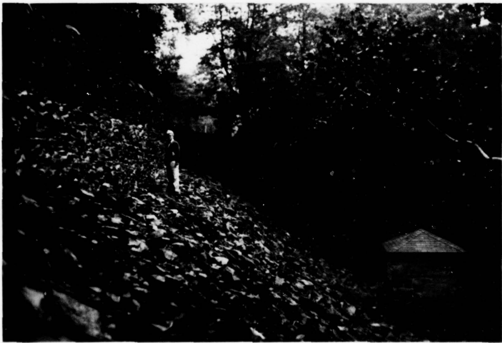
DAM, DOWNSTREAM SLOPE AND GATEHOUSE
