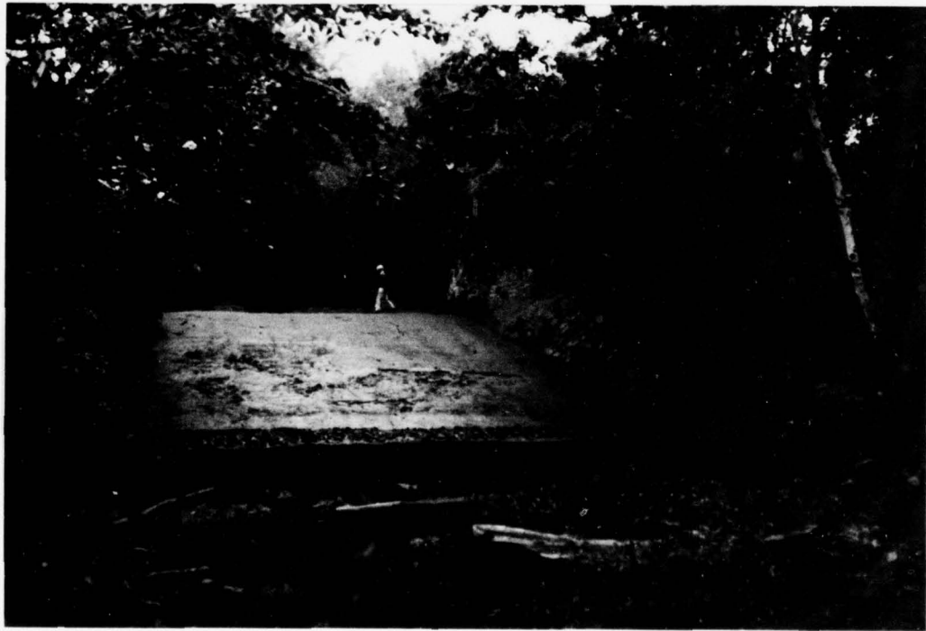
SPILLWAY EXIT, LOOKING UPSTREAM
