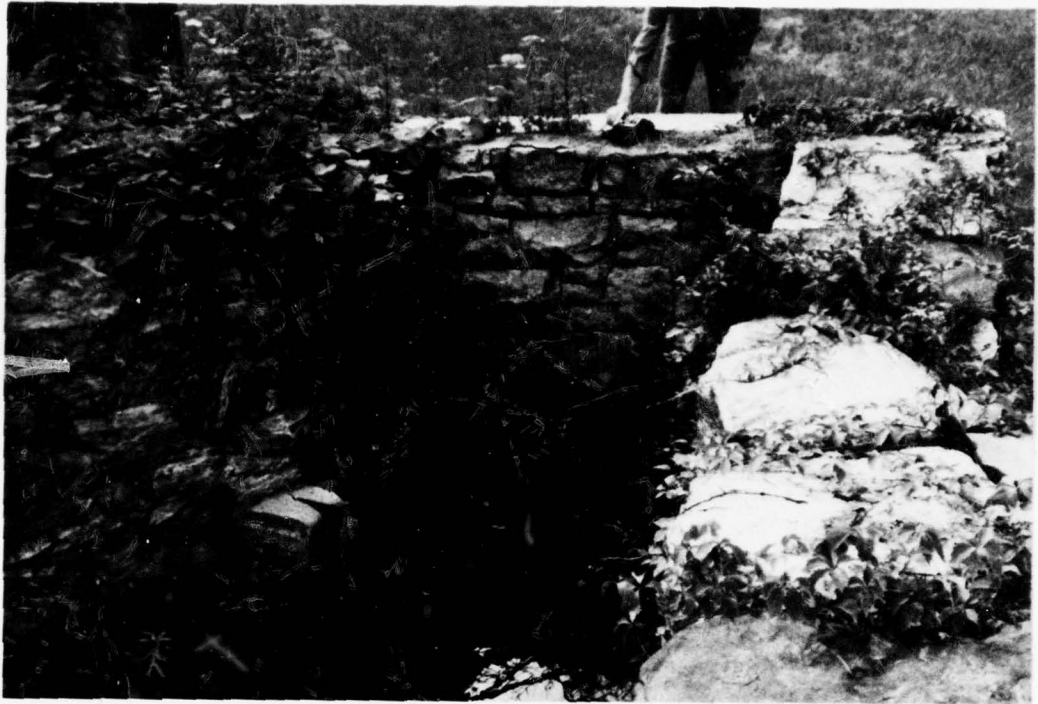
11) ENTRANCE OF CONDUIT, NOTE MEASURING WIER
