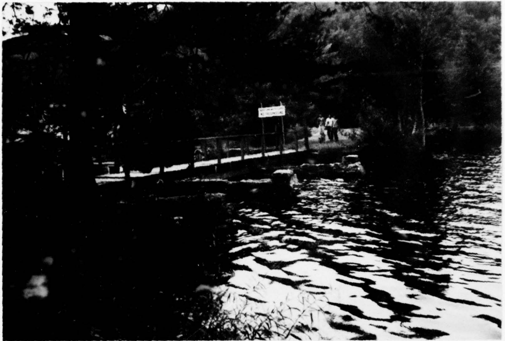
7) APPROACH CHANNELS TO SPILLWAY
