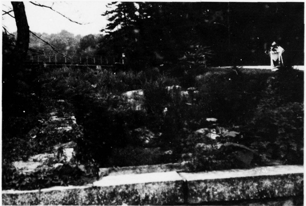
10) SPILLWAY CHANNEL LOOKING UPSTREAM
