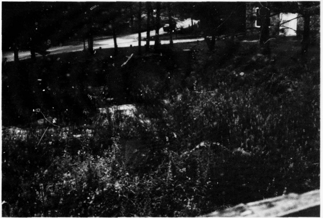
9) SPILLWAY CHANNEL LOOKING DOWNSTREAM, NOTE ENTRANCE OF CONDUIT AND HEAVY VEGETATION
