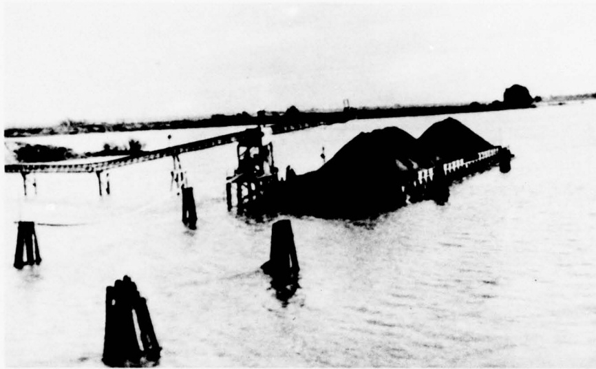
Figure 8. A 36-in. belt conveyor loading operation (photo courtesy of Sacramento District)
