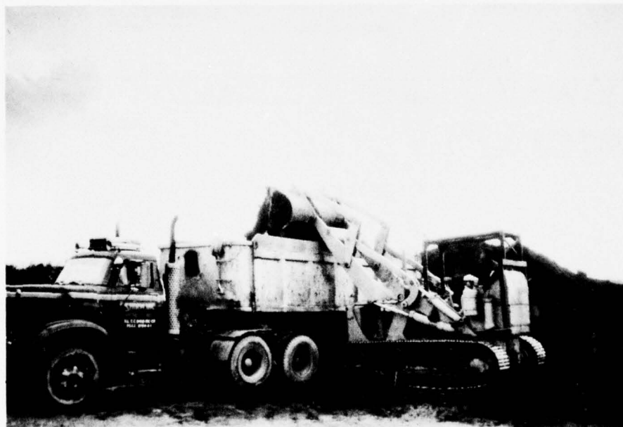
Figure B8. Loading dredged material at borrow area
