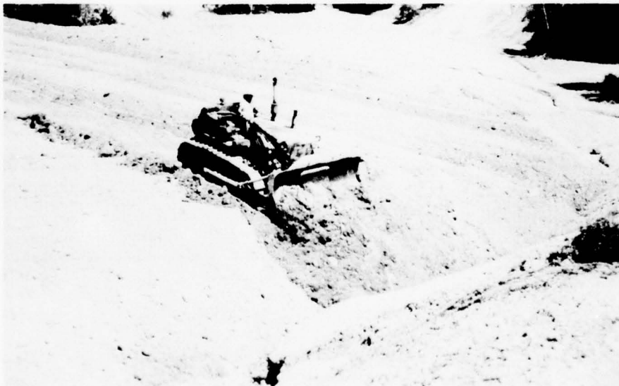
Figure 11. A bulldozer "striking off" the mine spoil ridges prior to covering with dredged material
