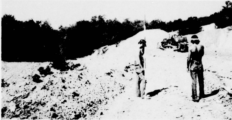
Figure B4. Leveling mine spoil ridges
