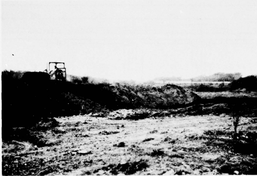
Figure B7. Stockpiling dredged material in borrow area
