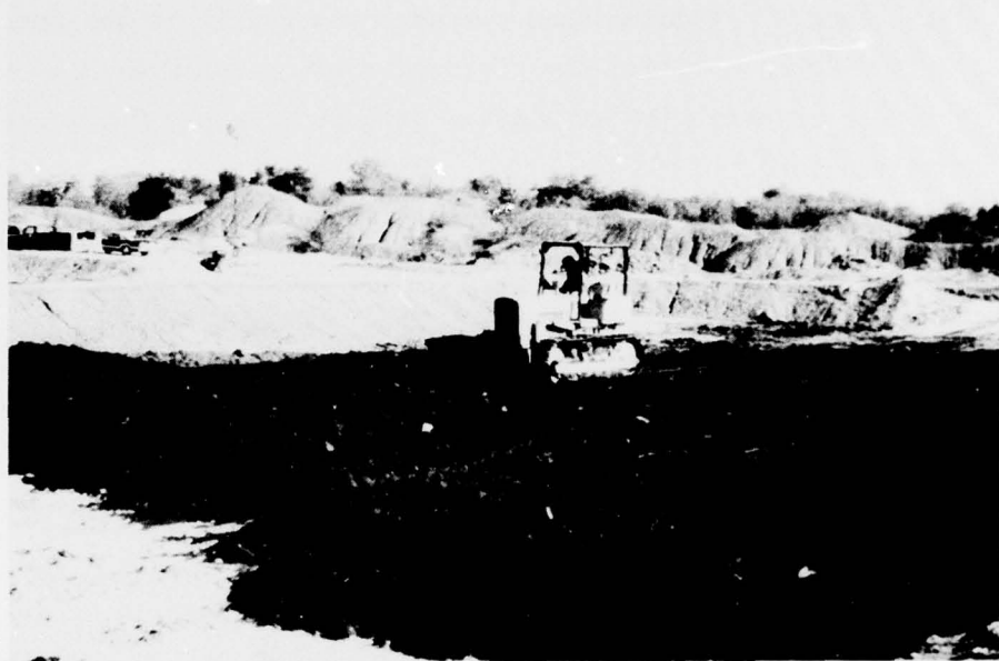
Figure B9. Spreading dredged material on plots
