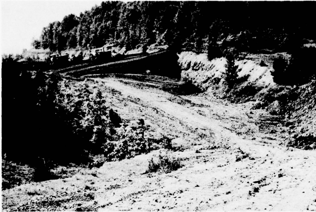
Figure 13. Backfilling of surface mined area (from McNay 35 )
