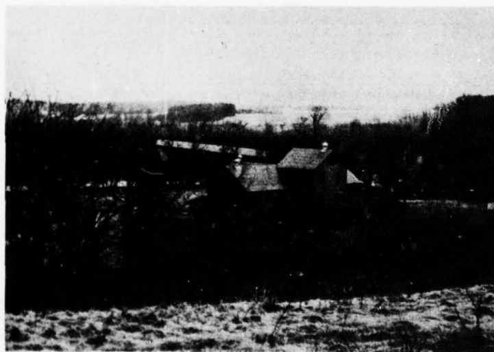
B) The Red Bridge Site from the Northeast
