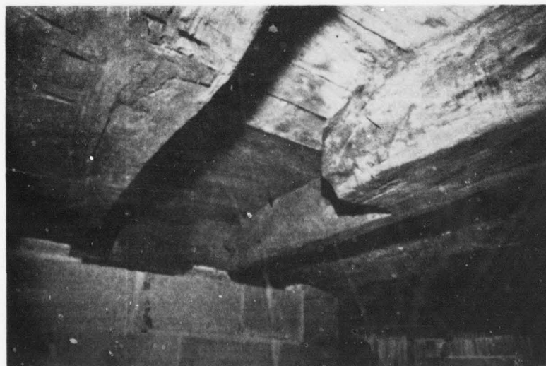
B) Cellar Room 001, First Floor Joist, Southeast Corner
