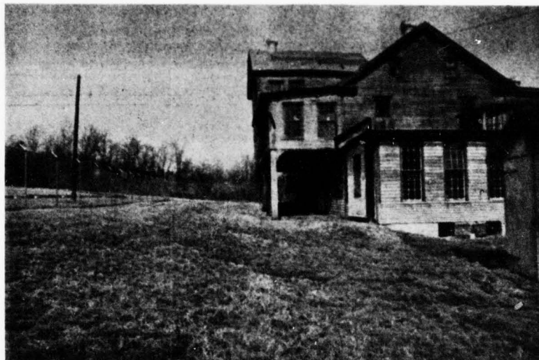
A) Northwest Corner of Structure Showing Existing Grading
