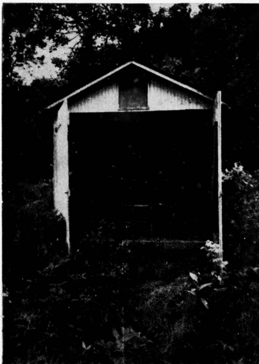
A) 1974 Iron Storage Shed
