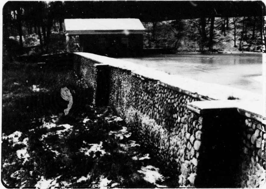
Downstream face of dam.
