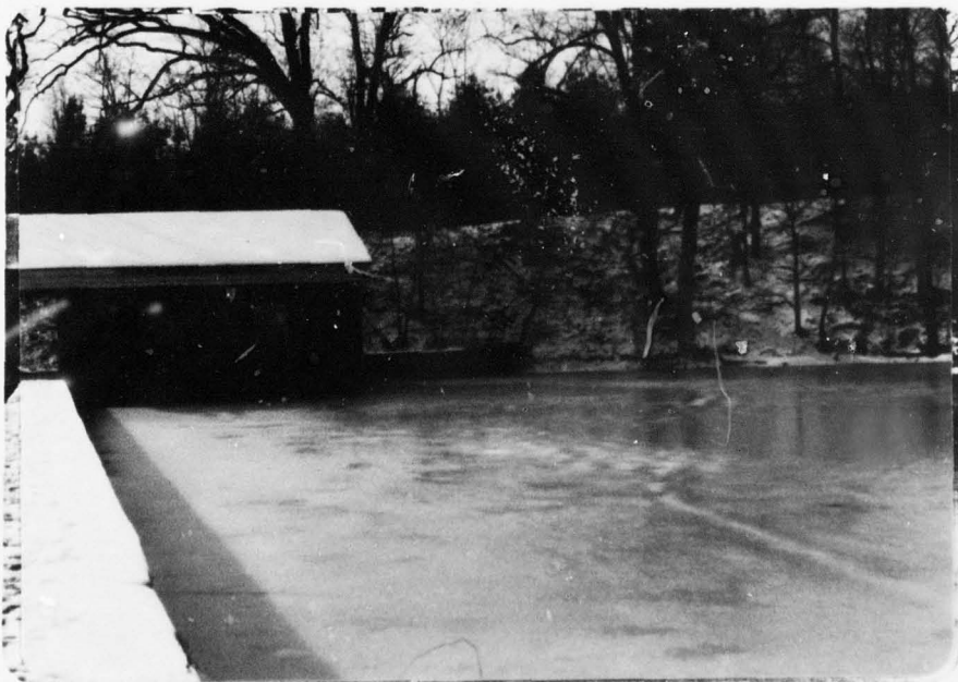
Right abutment. Looking South.
