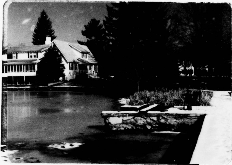
Discharge gate structure .
