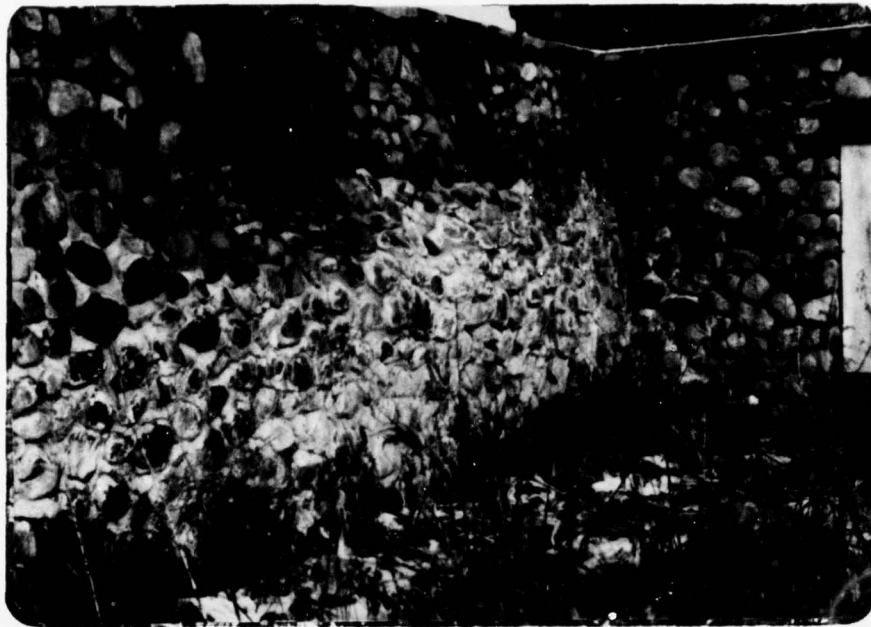
Bulging of lower portion of dam.
