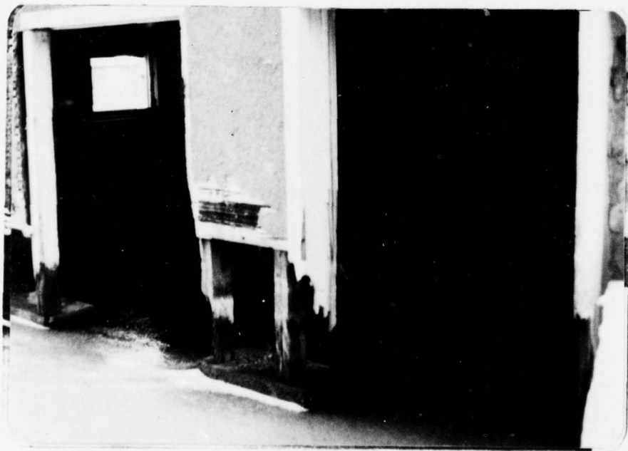
Abandoned boat house at right side of dam.
