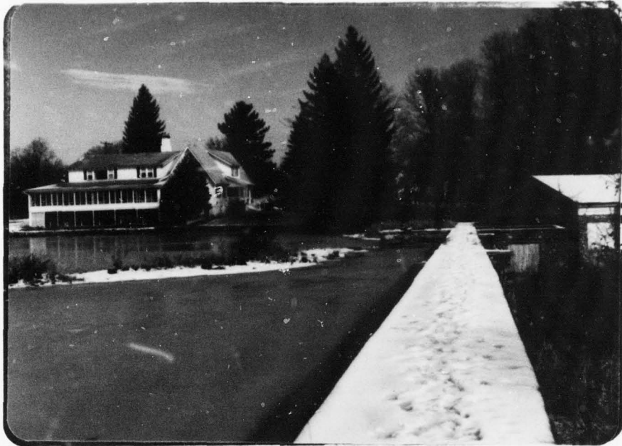
Crest of dam and left abutment. Looking North.
