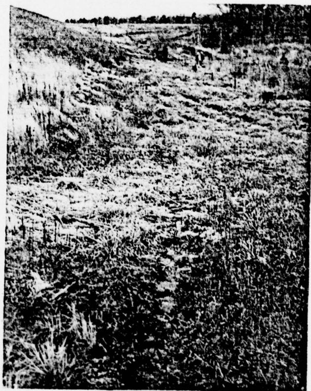
Seepage at downstream toe
