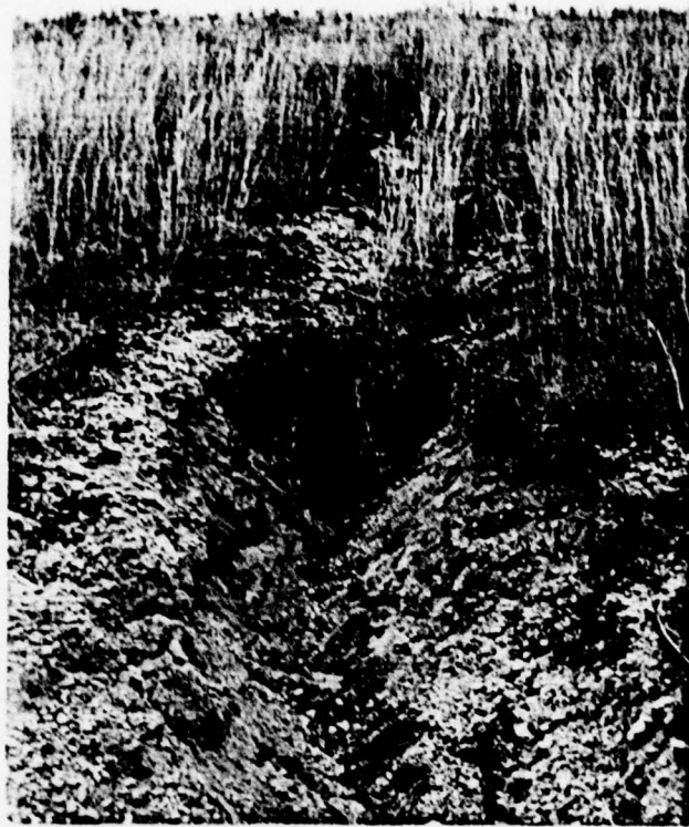
Erosion of downstream slope of dam
