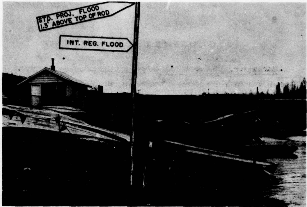
FIGURE 11 - Future flood heights at the confluence of the Moose and Kenai Rivers.
