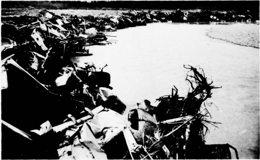
VIEW OF CAR BODIES USED FOR RIPRAP ON AN ERODING BANK
