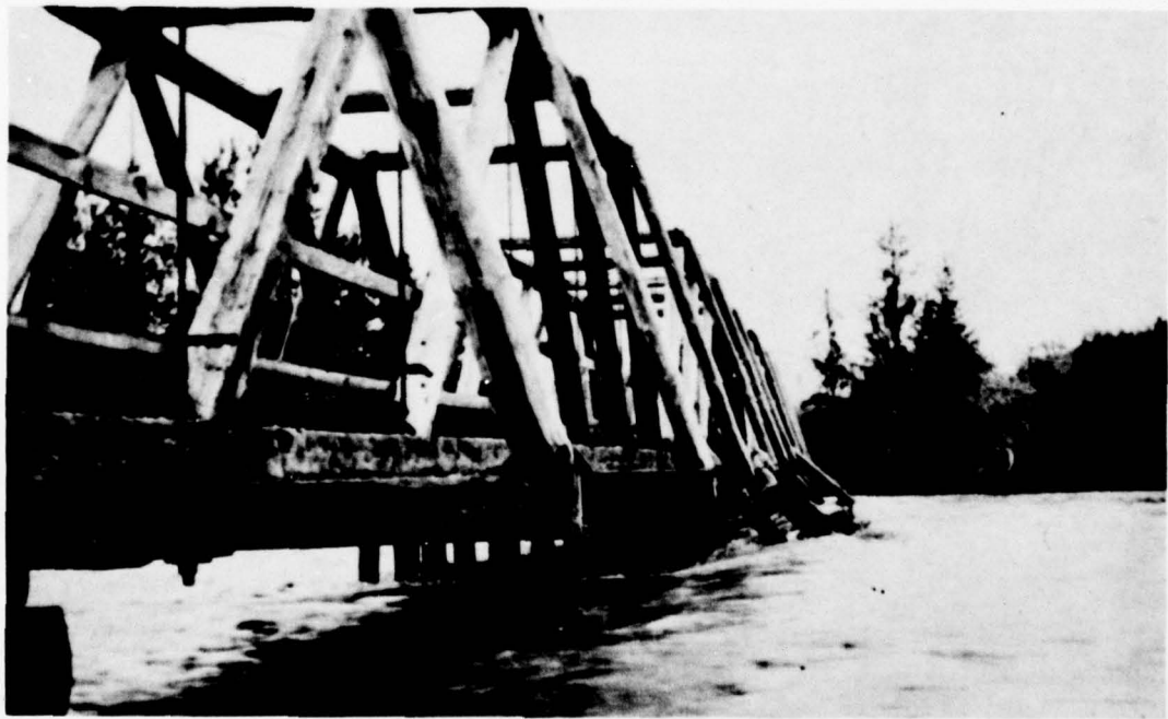
DEBRIS STARTING TO COLLECT AGAINST BRIDGE -FLOOD OF SEPTEMBER 1927
