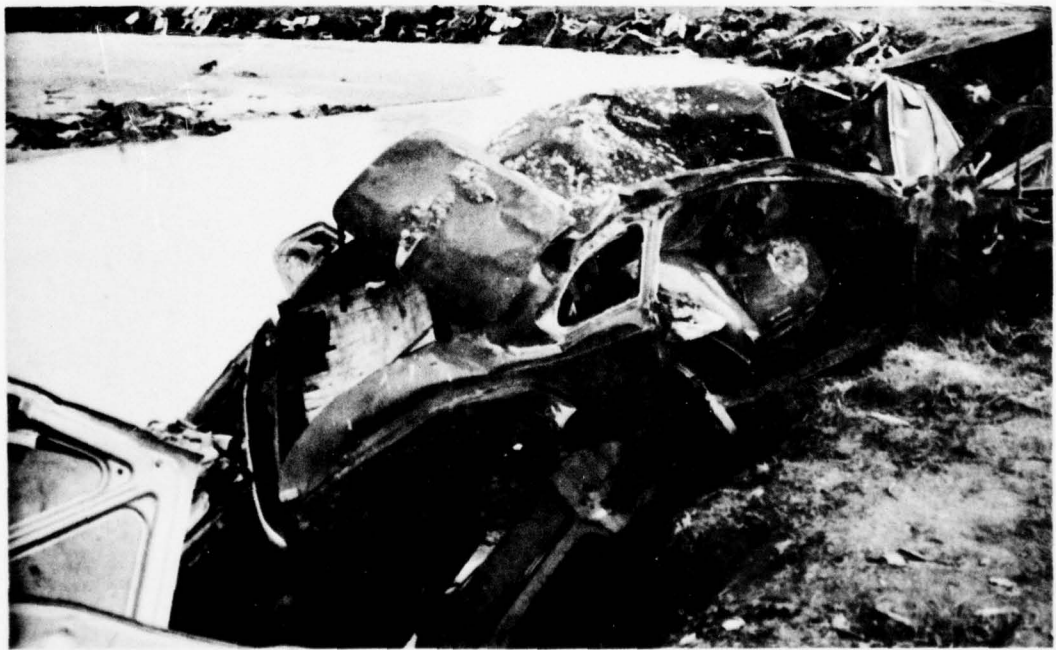
METHOD OF PLACING CARS WILL NOT STOP EROSION - IT DOES INCREASE FLOOD HAZARD
