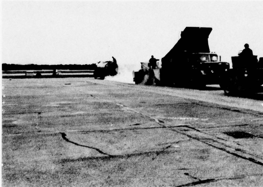
Photo 19. Fort Devens--placement of asphalt rubber and chips, and rolling of U. S. Rubber test area on apron
