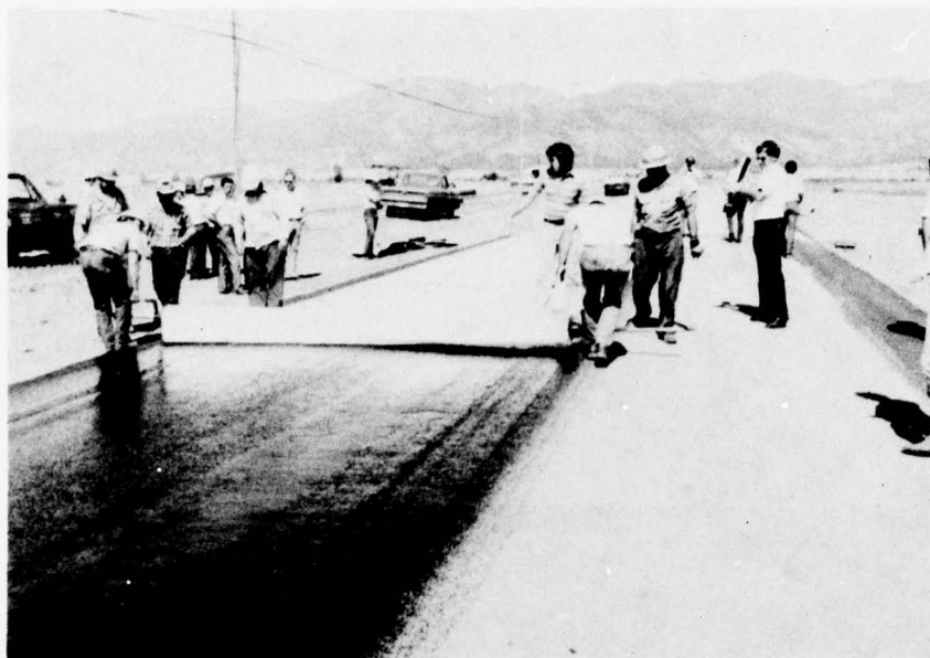
Photo 47. Fort Carson--placement of Mirafi 140 fabric
