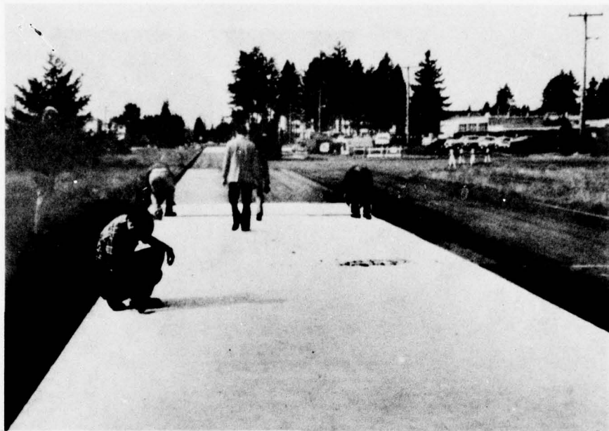
Photo 39. Fort Lewis--placement of Mirafi 140 fabric
