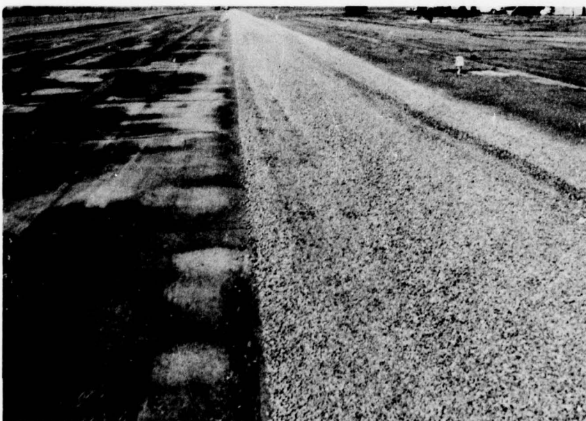
Photo 18. Fort Devens--asphalt rubber and chips after rolling
