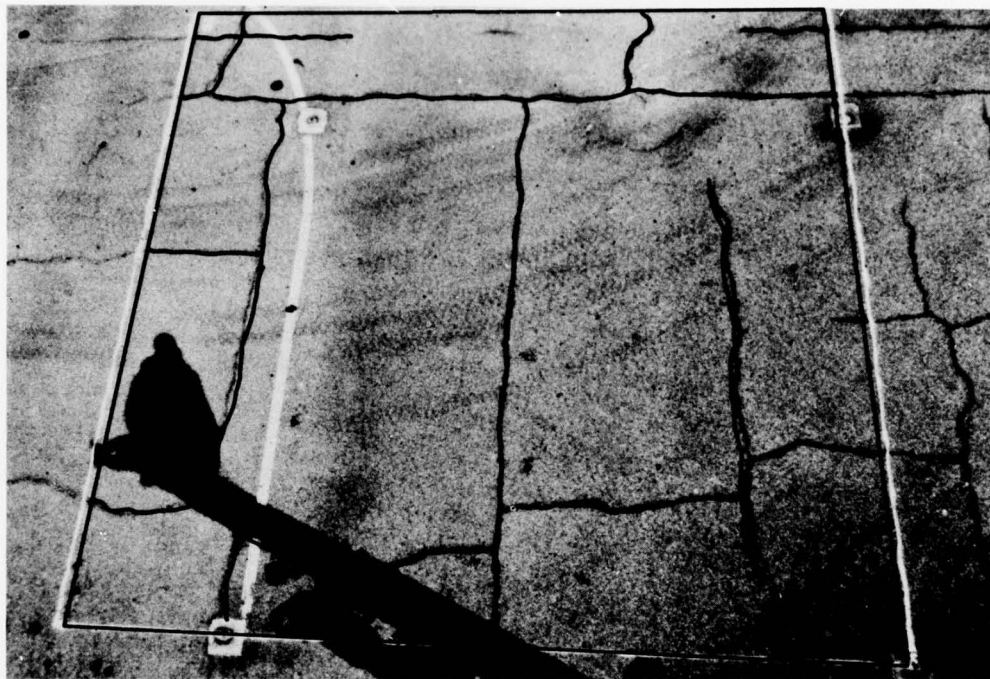
a. Condition of surface prior to overlay
