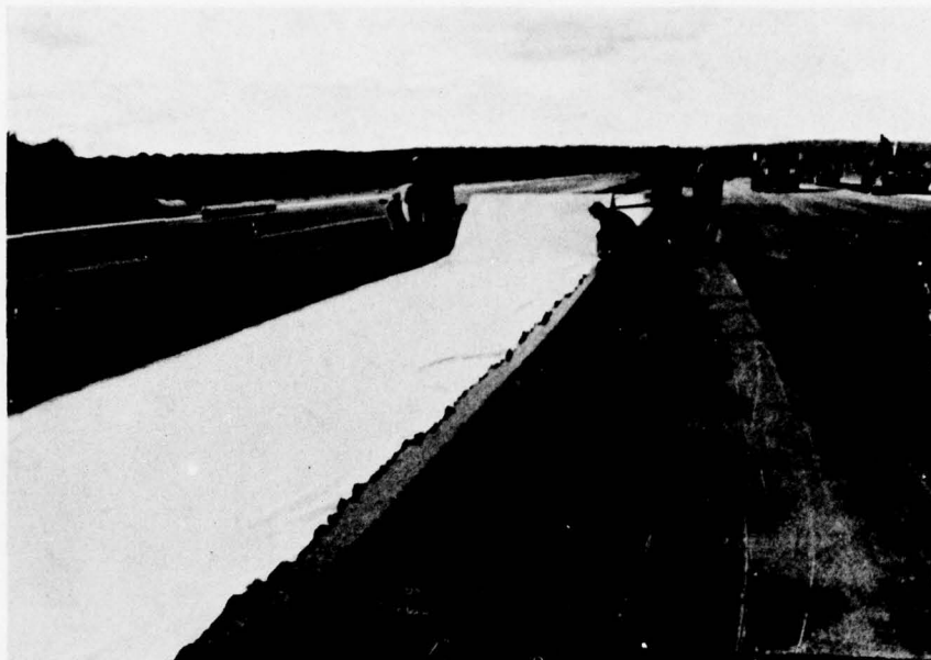
Photo 5. Fort Devens--sawed edge of Bidim C-22 gave a ragged appearance; material smoothed out under roller
