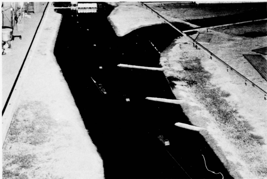
b. Leaving lock and proceeding upstream along left bank
