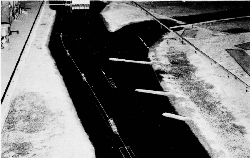
a. Approaching lock from along left bank with tow drifting from a considerable distance upstream of lock
