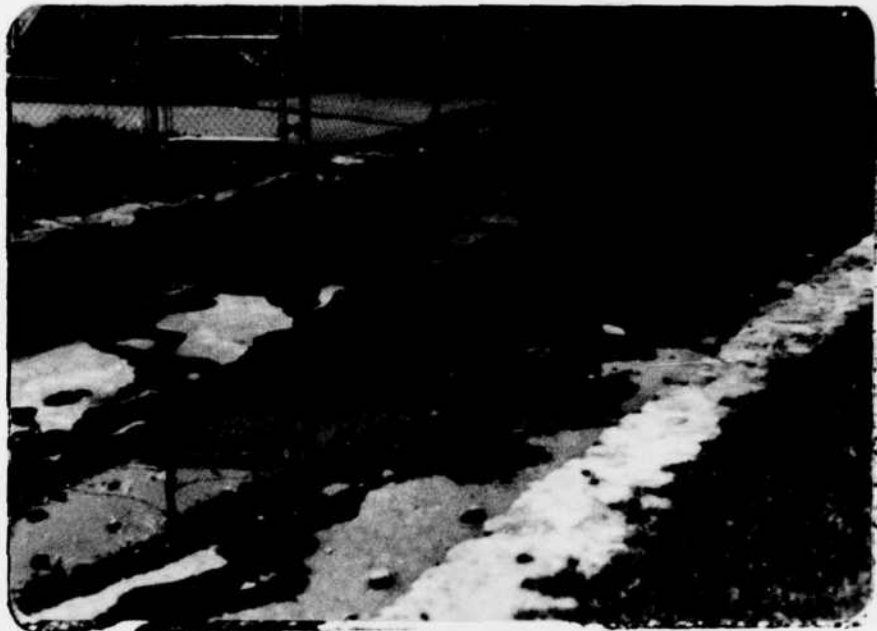
Deteriorated asphalt of discharge channel for fountain.
