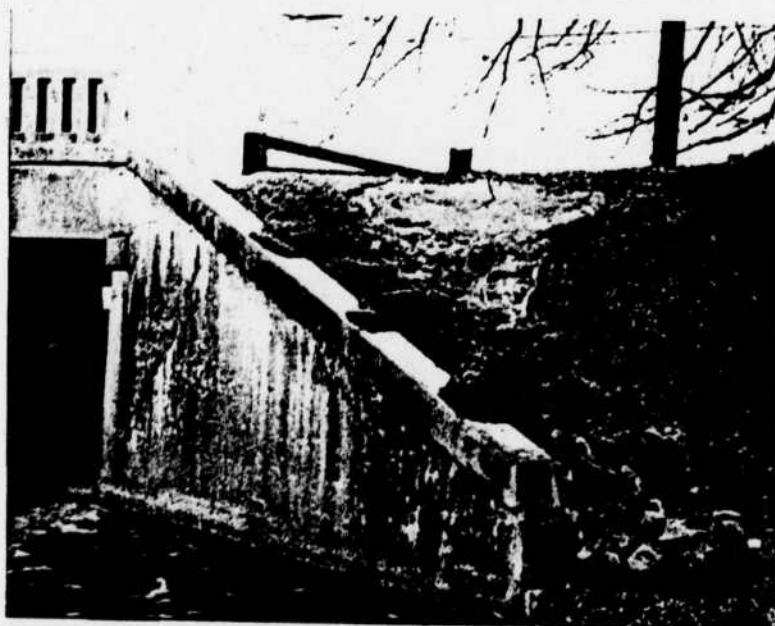
Downstream view of East abutment
