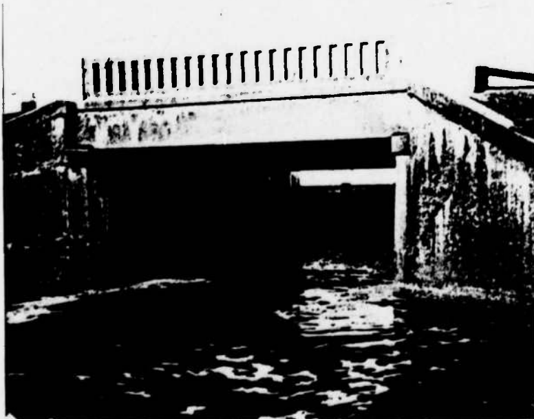
Downstream view of bridge and spillway
