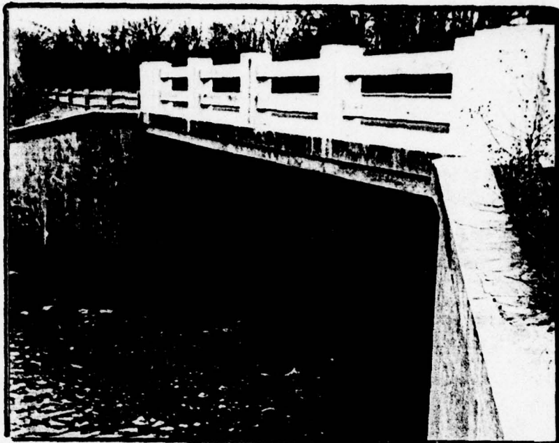
County bridge just below spillway
