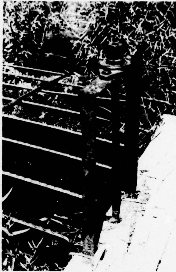
FIGURE 7 TURNING NUT AND RISER ROD FOR SLUICE GATE
