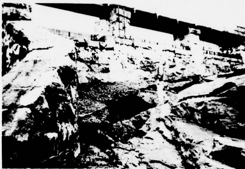
7. A closeup of the encircled eroded spillway channel area shown in Picture #6.
