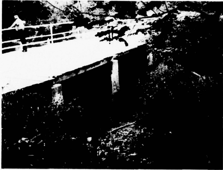
BRIDGE OVER SPILLWAY APPROACH
