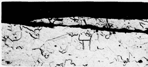
b) Joint interface at exterior showing lack of bond and tight crevice.
