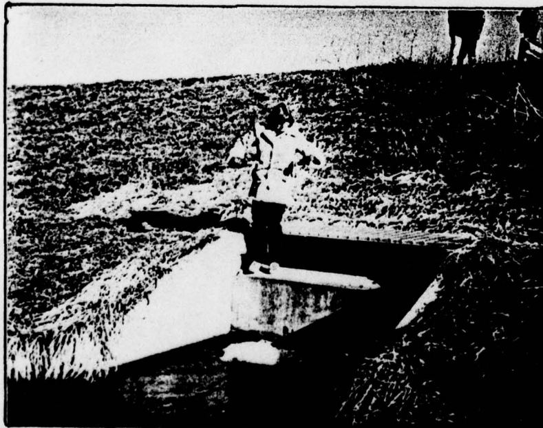
View of outlet structure
