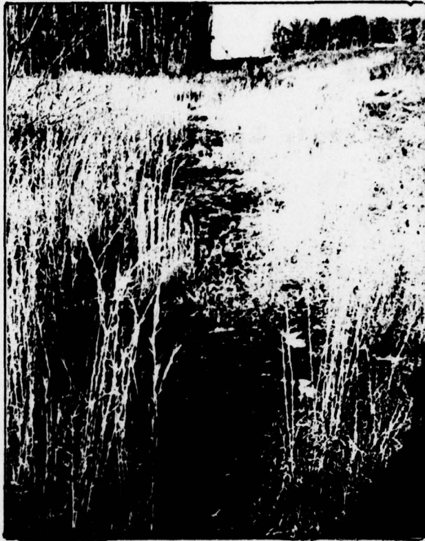
View of seepage at toe of embankment
