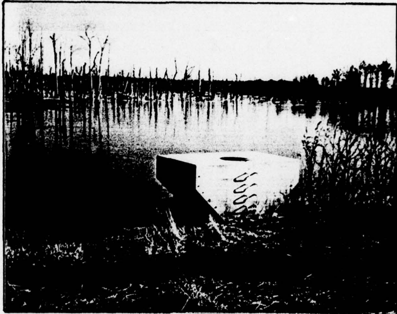
View of intake structure
