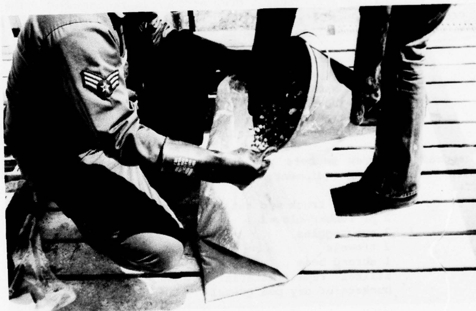
Figure 14 Adding Pea Gravel to the Mortar
