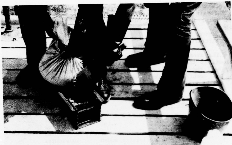
Figure 15 Slitting the Mixing Bag Open with a Trowel
