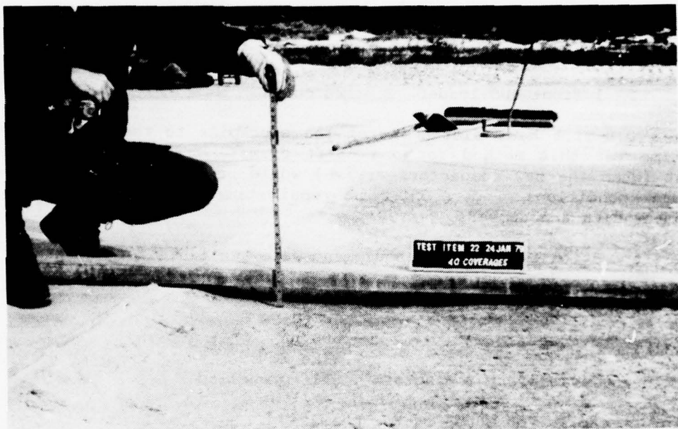
Figure 6 Consolidation of Crushed Stone at Edge of Concrete
