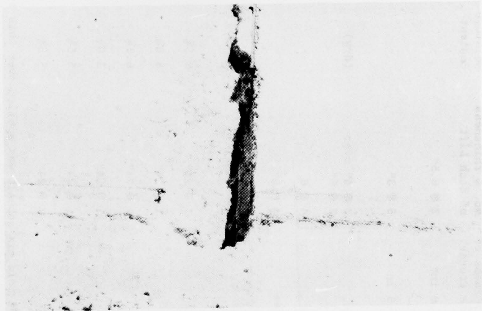
Figure 29 Spall at Small Crater Test Facility
