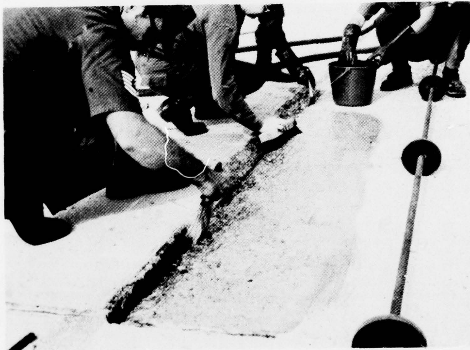
Figure 27 Primer Added to Insure Bond to Concrete to be Overlayed
