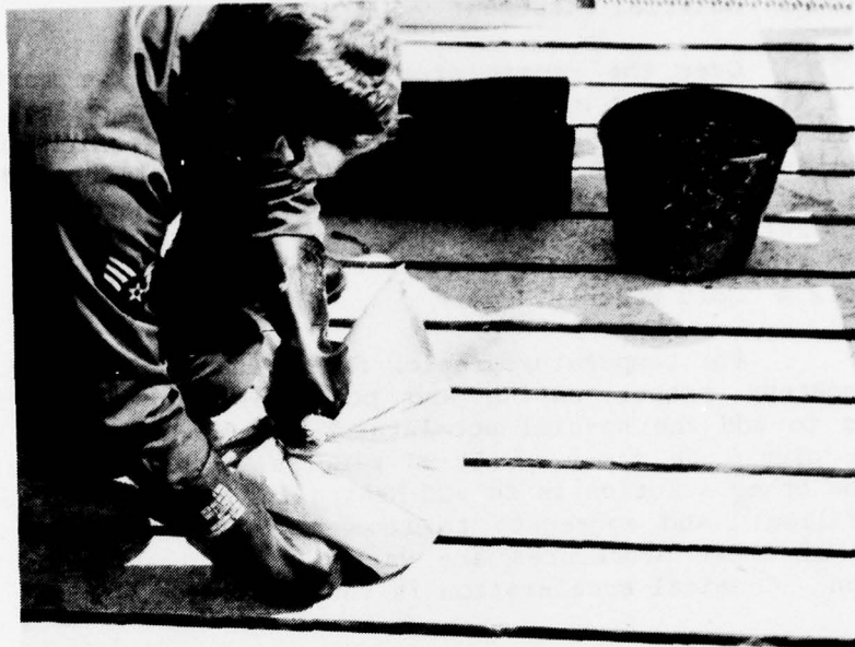
Figure 13 Thoroughly Mixing the Polymer Mortar
