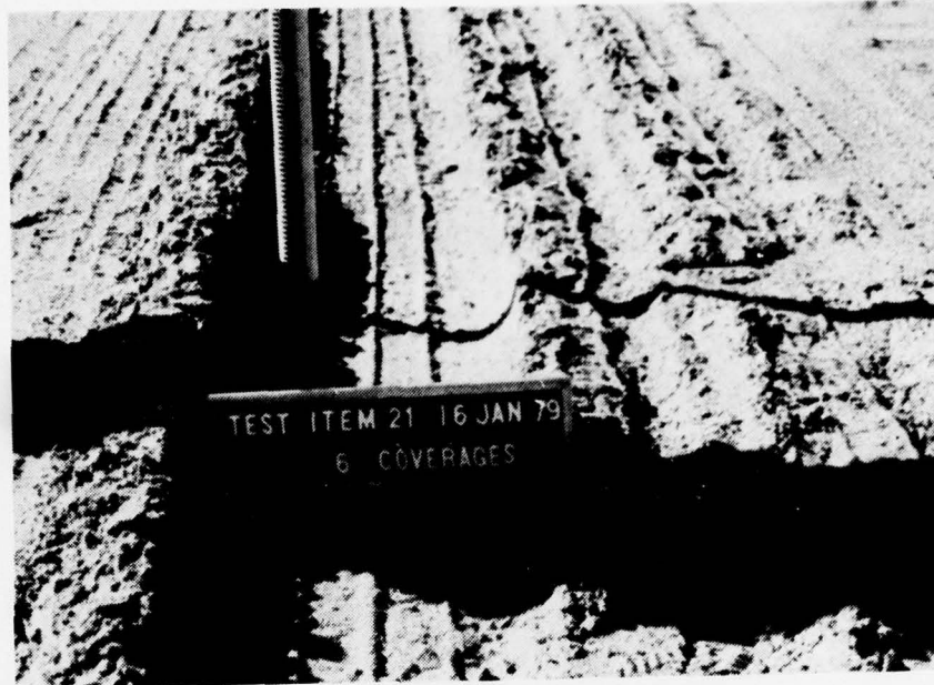
Figure 22 Actual Failure Due to Rutting
