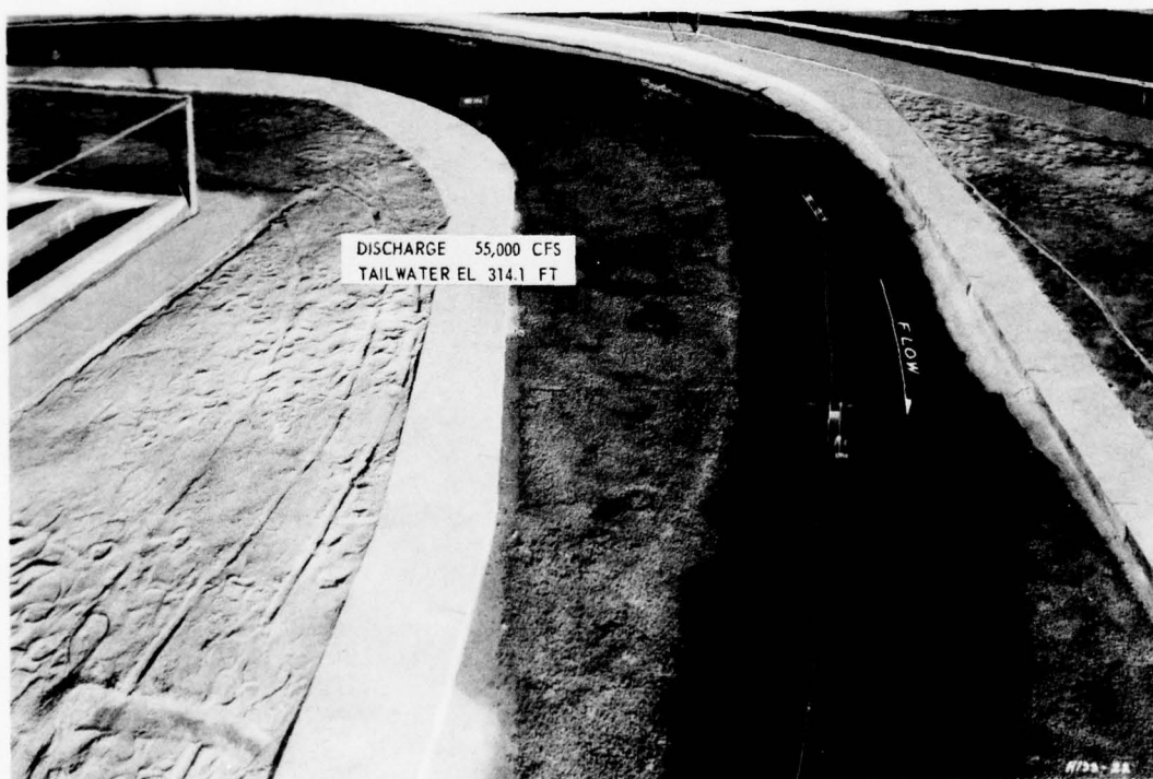
Photo 7. Existing conditions; path of upbound tow driving the bend at mile 25.6
