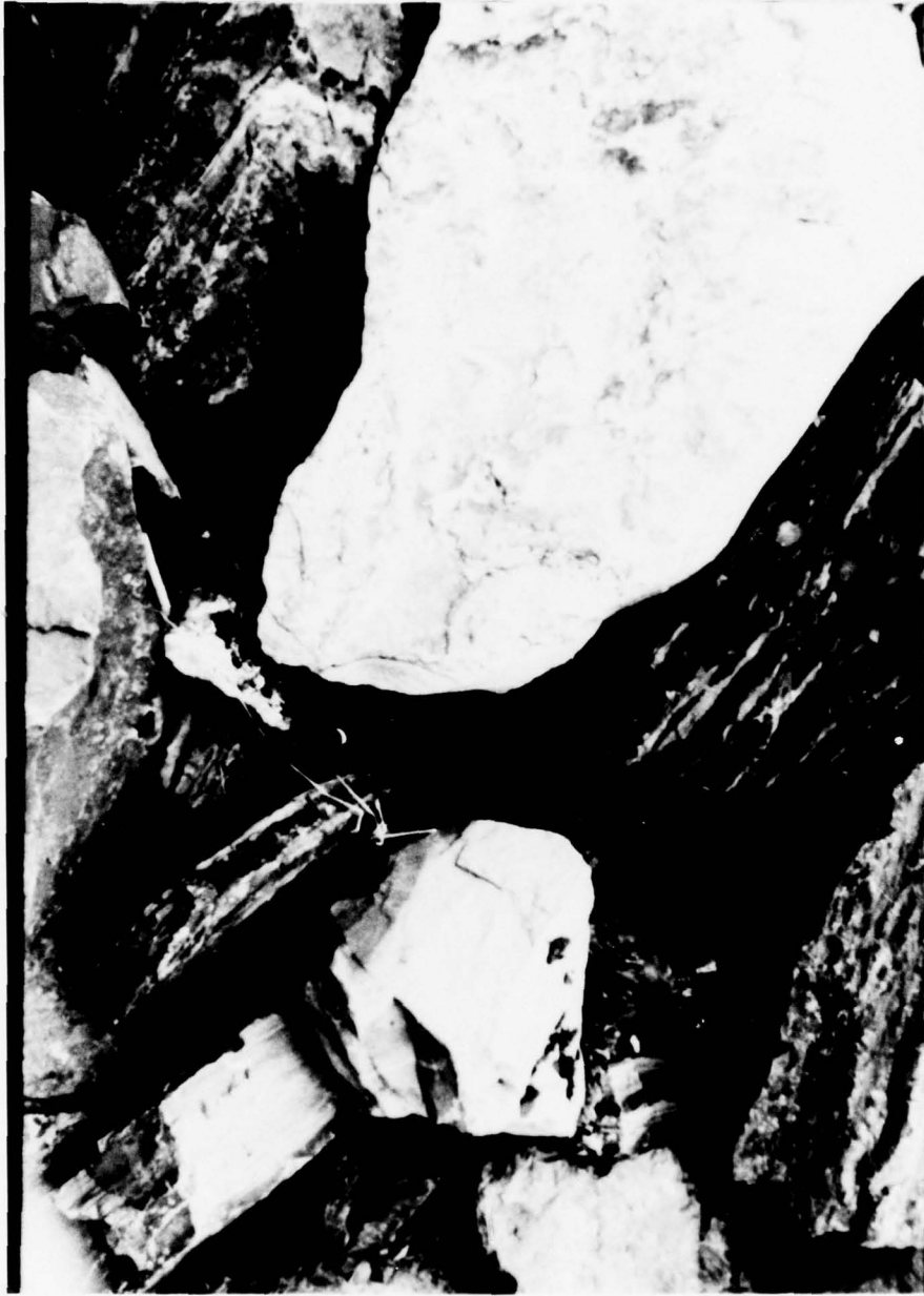
VIEW OF RIPRAP ON UPSTREAM SLOPE. NOTE FINE AGGREGATE FILTER LAYER BETWEEN RIPRAP.
