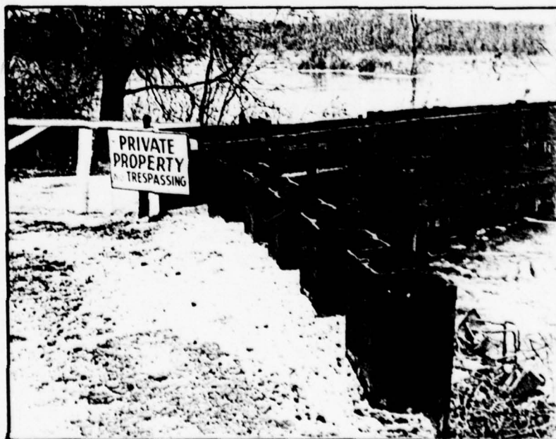
Steel sheeting at left spillway abutment
