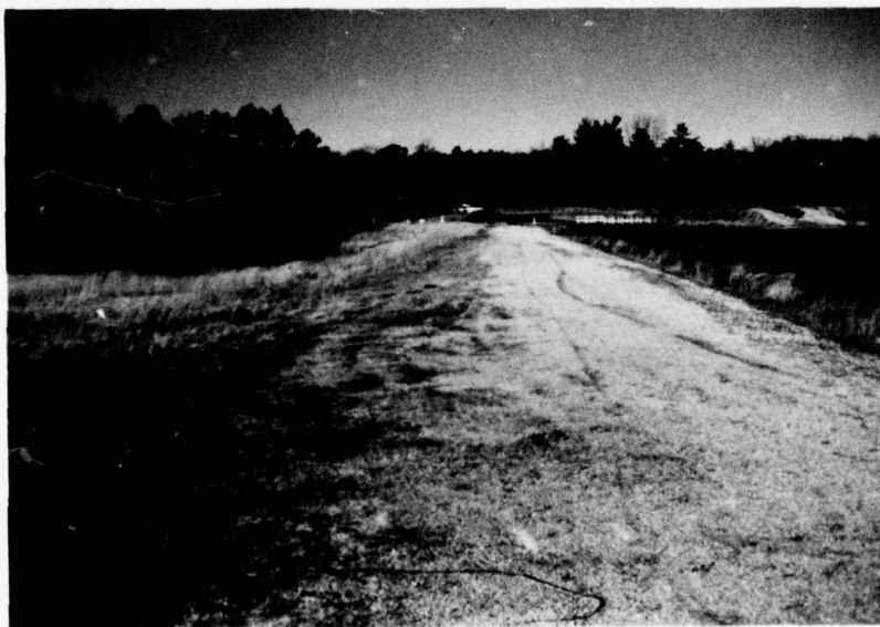
PHOTO 2 CREST OF DAM
