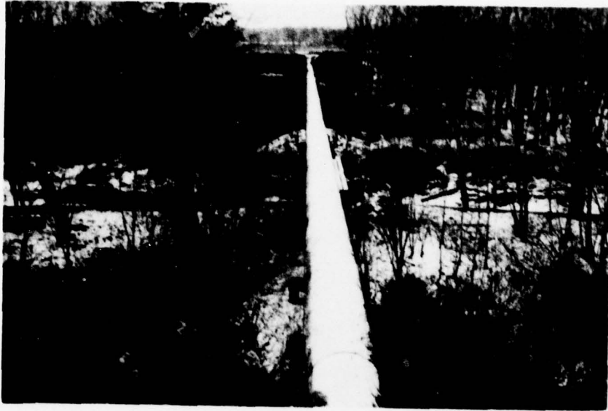
Photo 7 - Elevated portion of 48-inch transfer pipeline, looking toward Canoe Brook Reservoir No. 1. (11-29-78)
