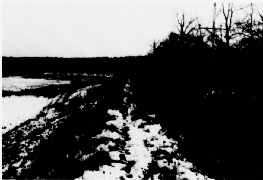
Photo 2 - Southern embankment, showing wave-cut inboard slope. (11-29-78)
