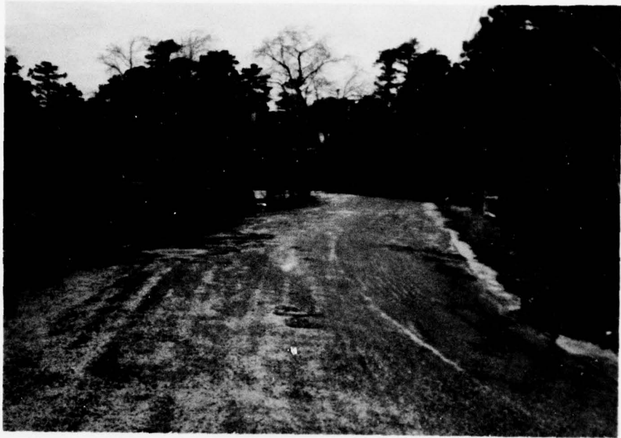
PHOTO 9 ROAD ON CREST OF DAM.
