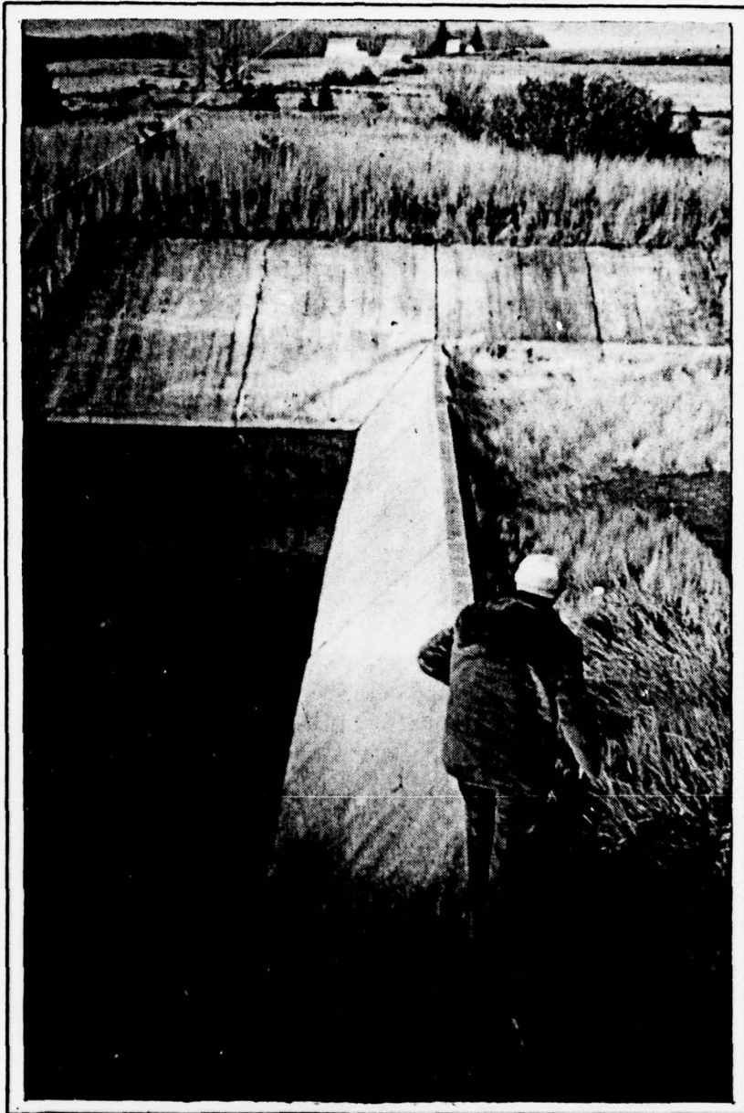
OVERVIEW OF TRAPAZOIDAL WEIR OF EMERGENCY SPILLWAY LOOKING TOWARDS RIGHT ABUTMENT.
