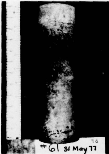
Figure B19. No. 61 before.
