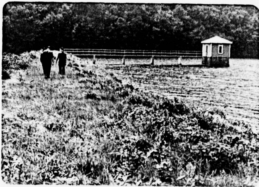
Photograph No. 3 Crest (looking south).
