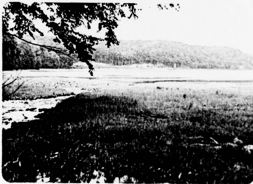
Photograph No. 10 Downstream: Lower Dam.
