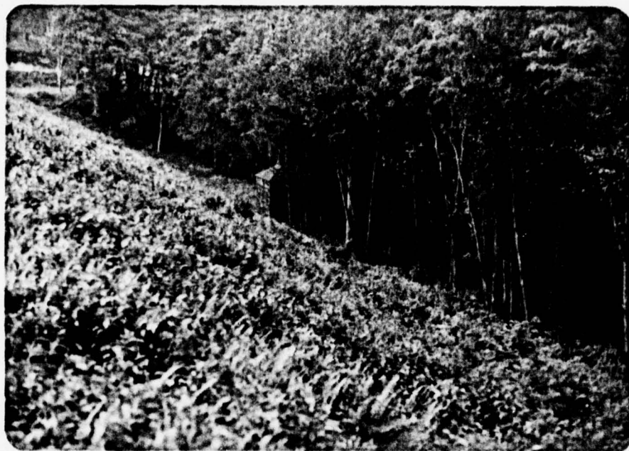
Photograph No. 7 Valve house.
