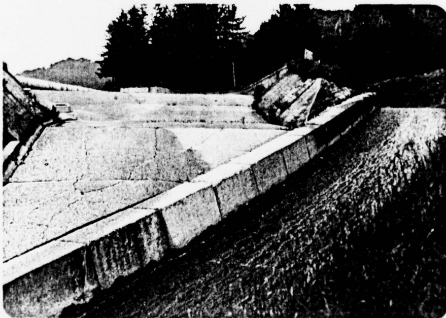
Photograph No. 4 Spillway chute.
