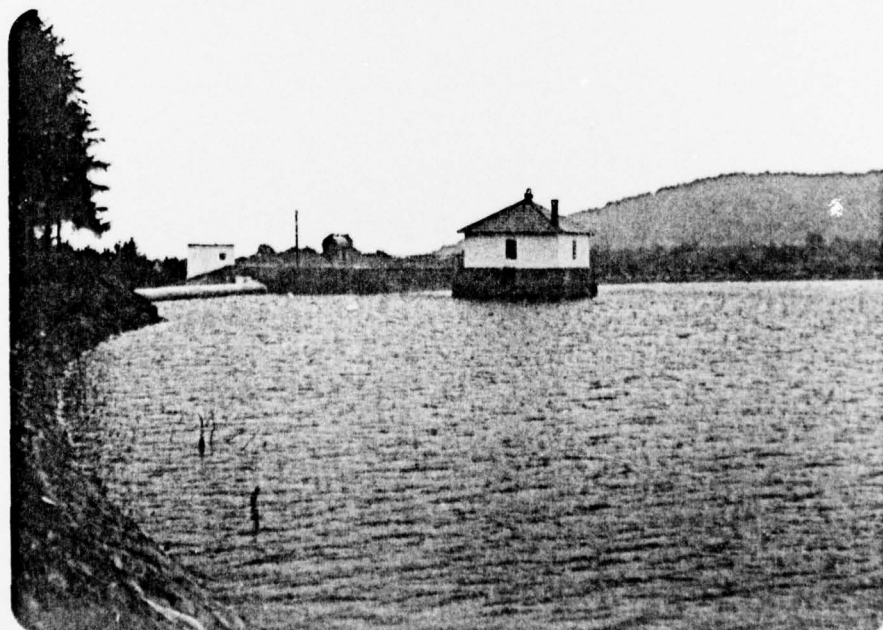
Photograph No. 2 Intake tower and spillway entrance.
