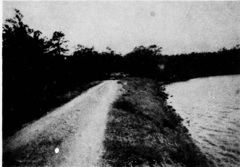
C. Right Abutment Area.
