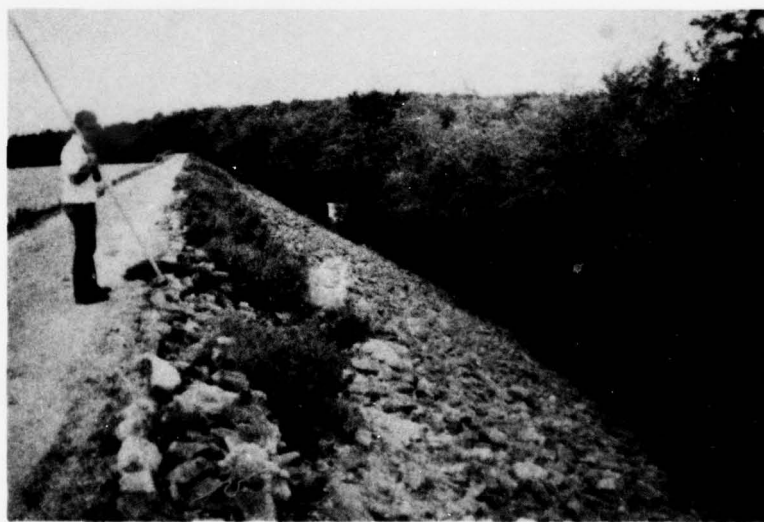
B. Downstream Slope of Embankment. View Toward Left Abutment.
