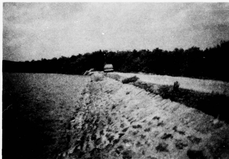
A. Upstream Slope of Embankment. View Toward Left Abutment.
