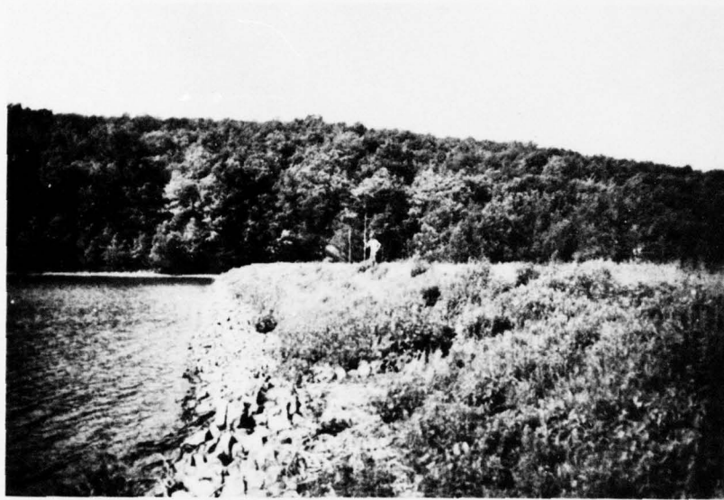
A. Upstream Slope of Embankment.
