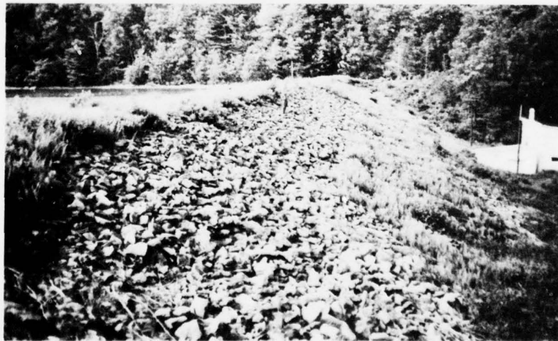
B. Downstream Slope of Embankment.
