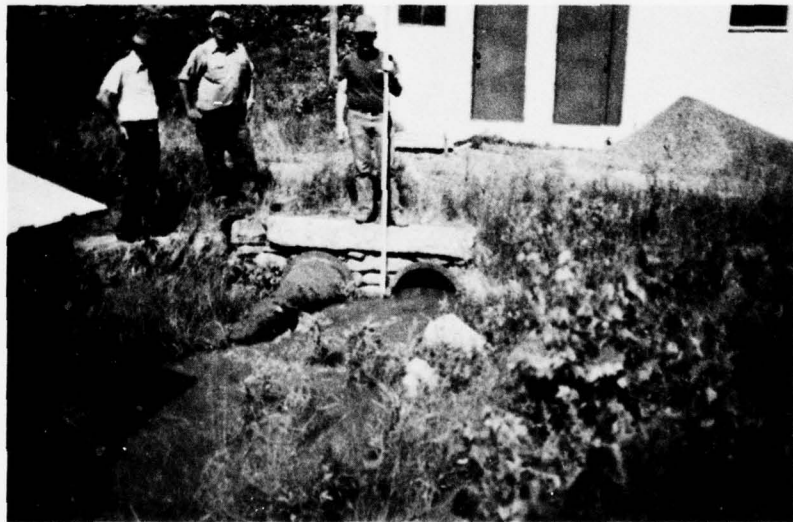
P. 20-Inch Blowoff During Operation.
