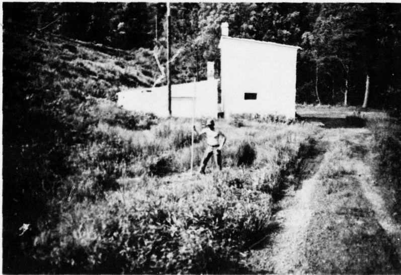
F. Wet Area at Toe 50 Feet Right of Gatehouse.
