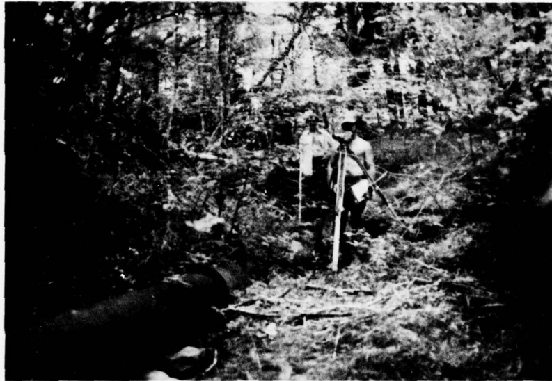
O. Excavated Area Between Diversion Channel and Original Channel of West West Branch Schuylkill River. View from Diversion Channel.
