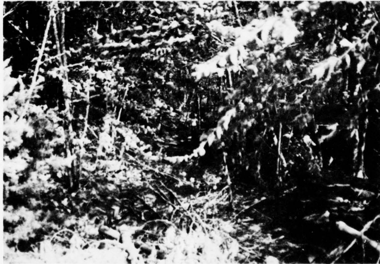
H. Right Spillway Discharge Channel.
