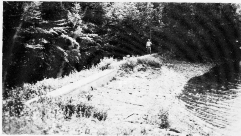
D. Right Spillway — View from Downstream.
