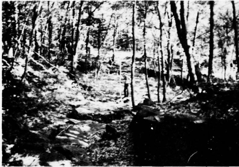
G. Left Spillway Discharge Channel.
