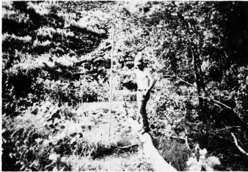
E. Wet Area at Toe Near Left Abutment.
