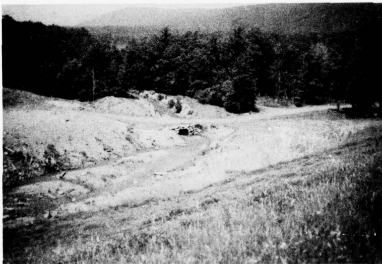
O. Downstream Channel Area.
