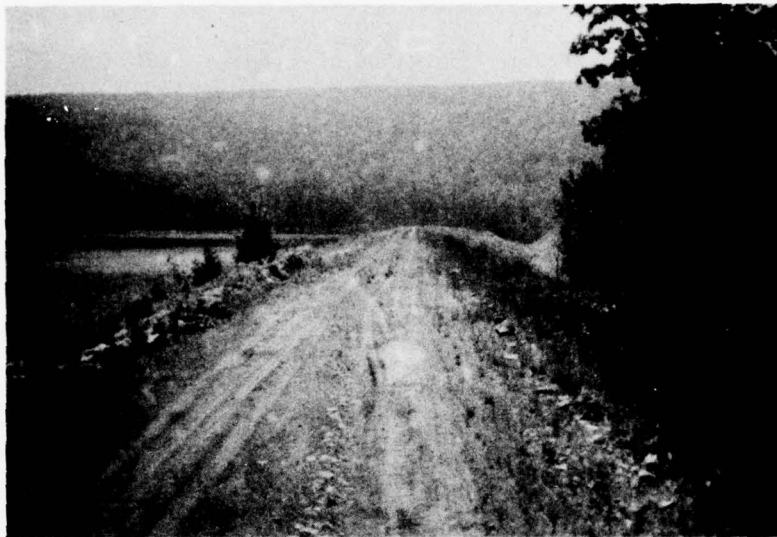
A. Embankment — View from Right Abutment.
