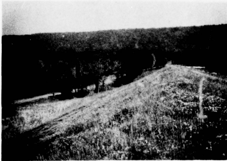
C. Downstream Slope of Embankment — View from Left Abutment.
