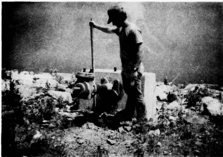
L. Gate Stand on Top of Dam.
