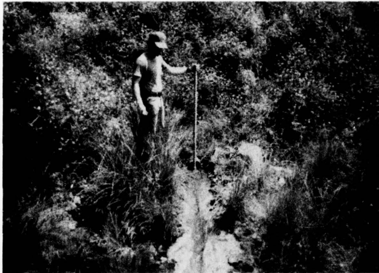
J. 6-Inch Toe Drain Outlet 400 Feet from Right Abutment.
