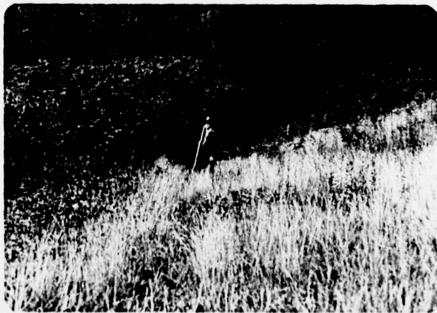
Photograph No. 6 High brush on downstream slope.
