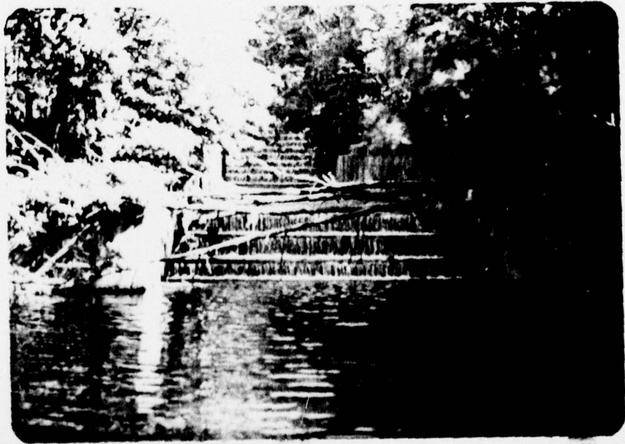
Photograph No. 4 Spillway discharge channel.
