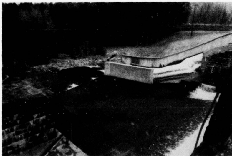
F. Concrete Apron of Masonry Gravity Spillway and Downstream Channel
